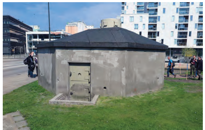
World War II machine-gun pillbox in Malmö, renovated and specially opened for us by local enthusiast Torbjörn Anderson. The observation tower can be seen on top
